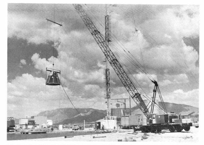
A NOSE CONE for the space shuttle's recoverable rocket boosters is readied for testing at Sandia's new Water Impact Target in Area III. The new facility is an extremely versatile tool for determining how objects survive high-speed impacts into water.
